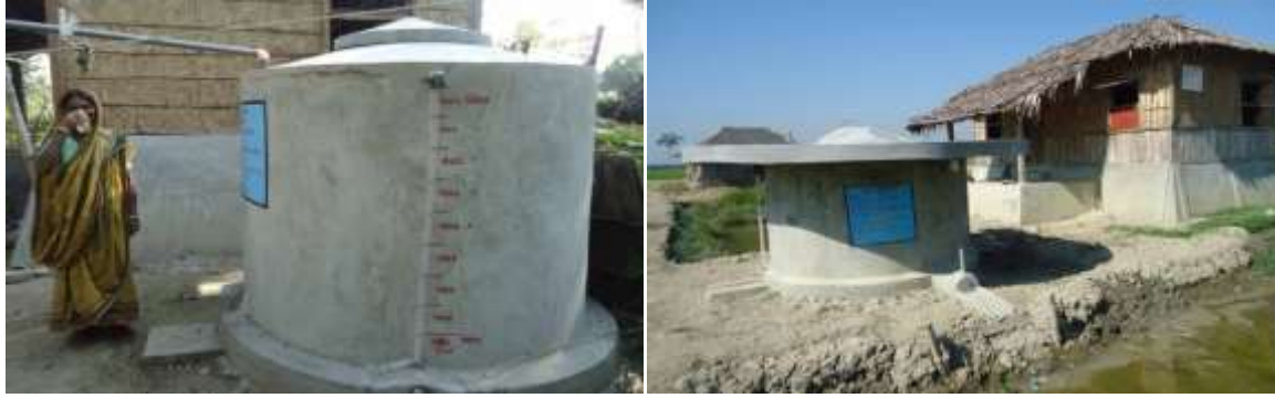
Figure 6: Ferro-cement (left) and brick-made (right) rainwater reservoirs of 3,200 and 3,600 L capacity respectively
