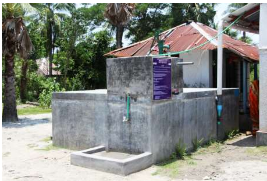
Figure 10: Community scale rainwater harvesting system in Bagerhat near a temple
