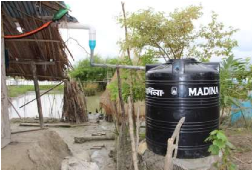
Figure 7: Household rooftop rainwater harvesting system of 1,000 L capacity in Satkhira
